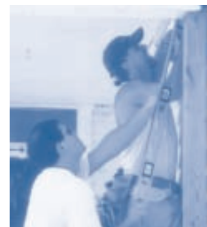
NeighborWorks® Week volunteers repair the porch of a homeowner in Gaston, Indiana.
