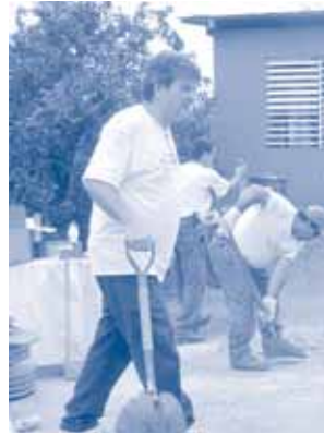
ROI staff, board members and volunteers cleaned and painted the La Casa de la Cultura in Castañer, Puerto Rico.
